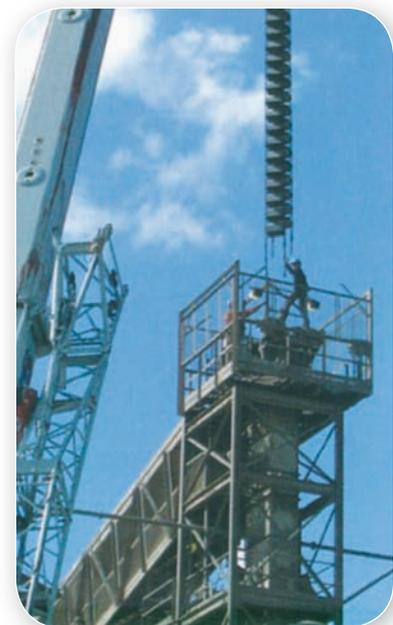
Quick and simple assembly of an endless chain strand
